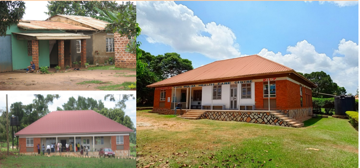
The original storefront Masooli clinic (top left), Faith Mulira Health Care Centre at its dedication in October 2008 (bottom left) and today, with its remodeled entrance and signage and (inside) expanded inpatient and surgical facilities.
